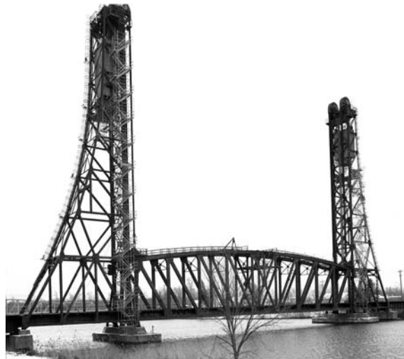
Welland Canal Lift Bridge Stair Towers
