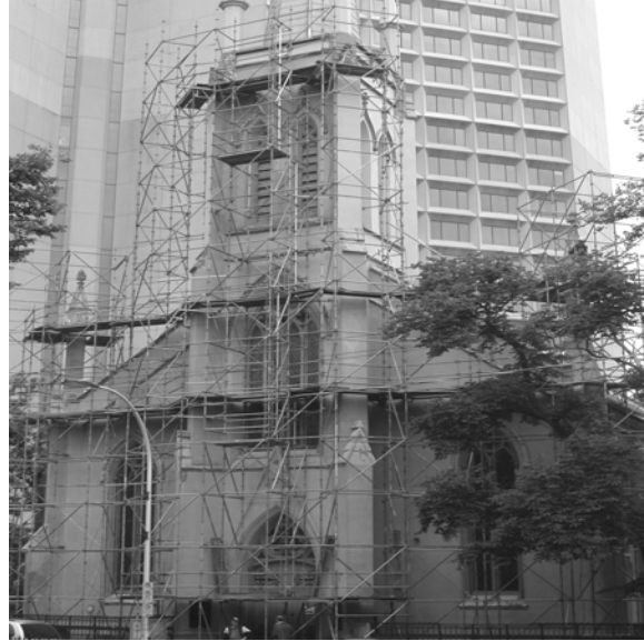
St. Matthew's Church, Halifax N.S. Scaffold Application
